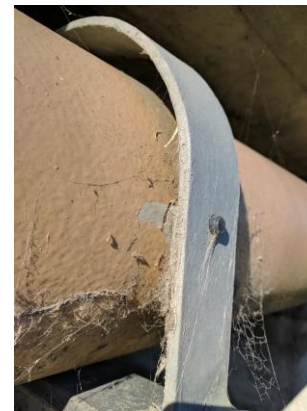
Figure 8: Ngaruroro Bridge Bracket Replacement
