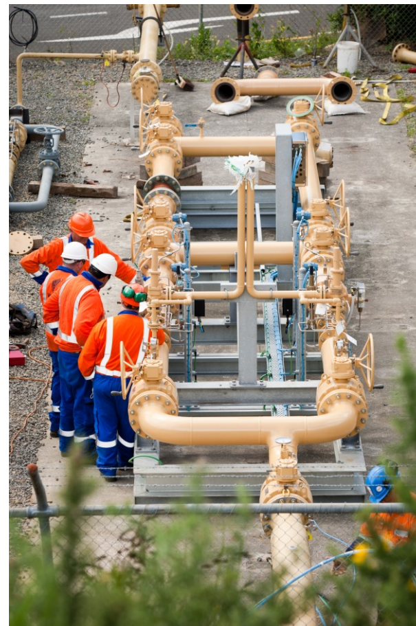
Figure 6.4: Tawa Gate Upgrade to Maintain Quality of Supply in Wellington (2011).
