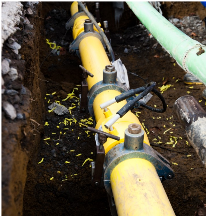
Figure 5.6: Electrofusion Operation to Joint Two Pipes.
