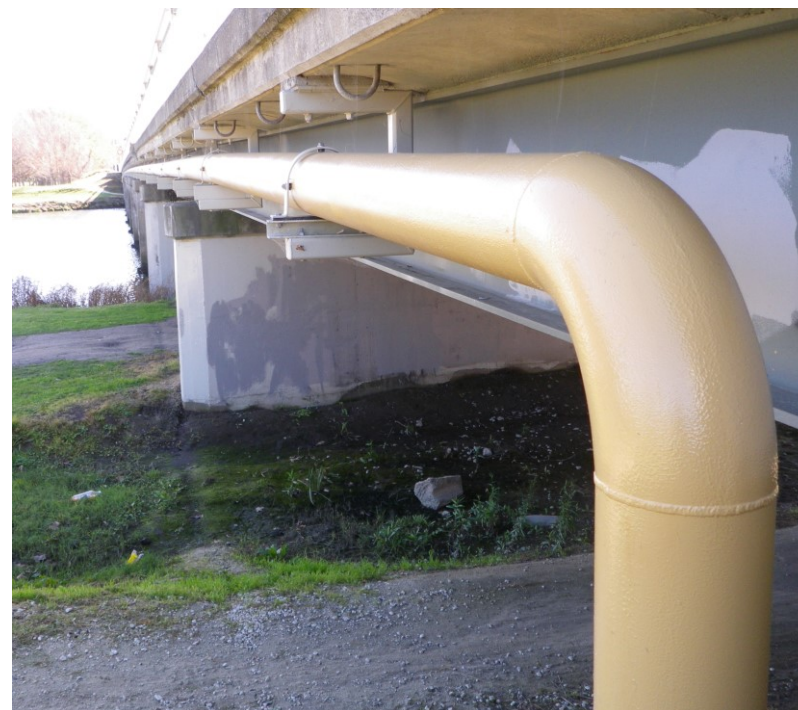
Figure 7.2: Bridge Crossing in Hawkes Bay
