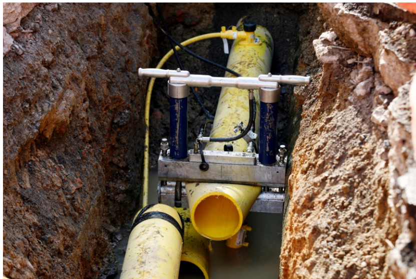
Figure 6.3: Pipe Repair Operation with Squeeze-off Equipment.
